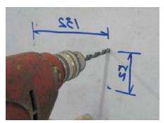
Pic18: drill the plastic expand hole
