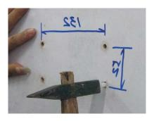
Pic19: knocking the plastic expand bolt
