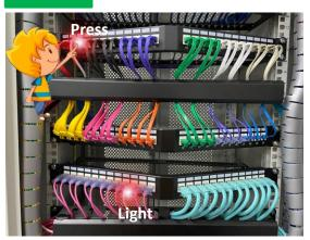
Simply press at either ends of the cable, both LED will illuminate at both ends.
